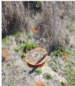
Manhole perimeter marking
