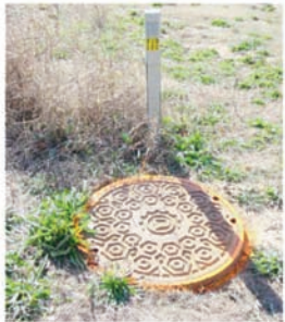
Manhole cover marking
