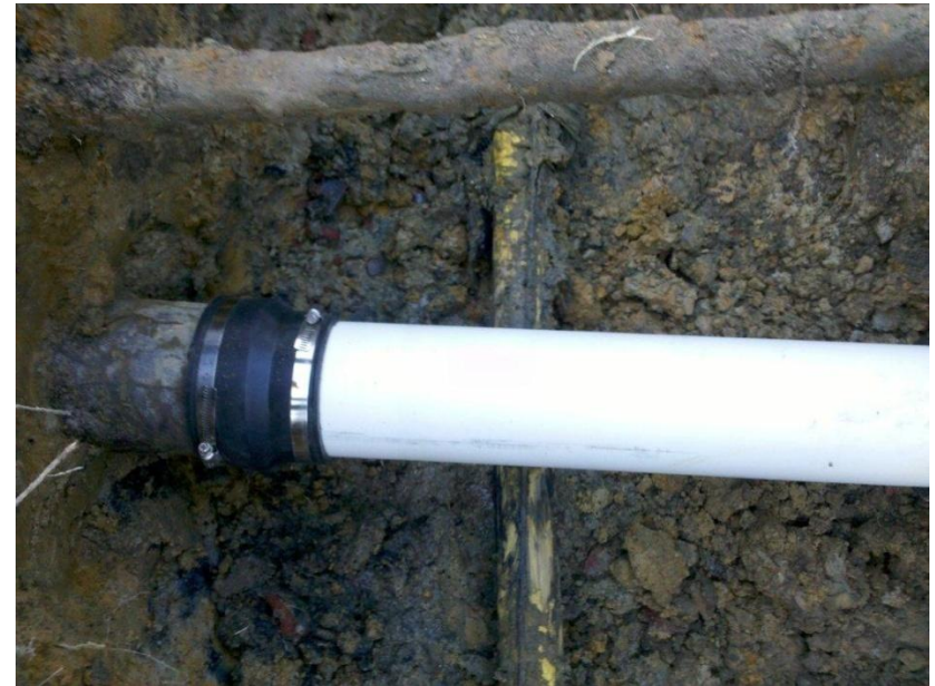
CROSS BORE AFTER REPAIR
